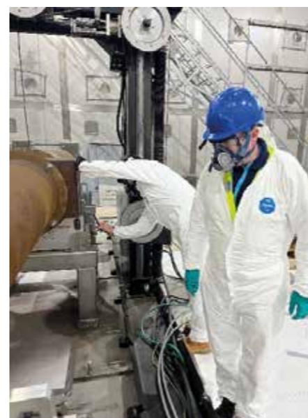
Checking cut progress during SAT
