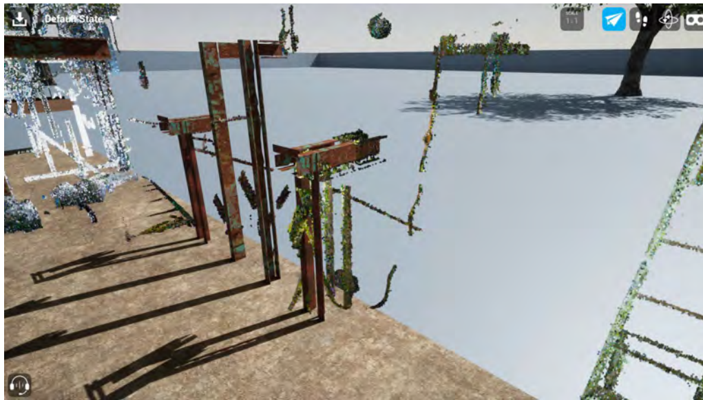
VR-enabled decommissioning site
